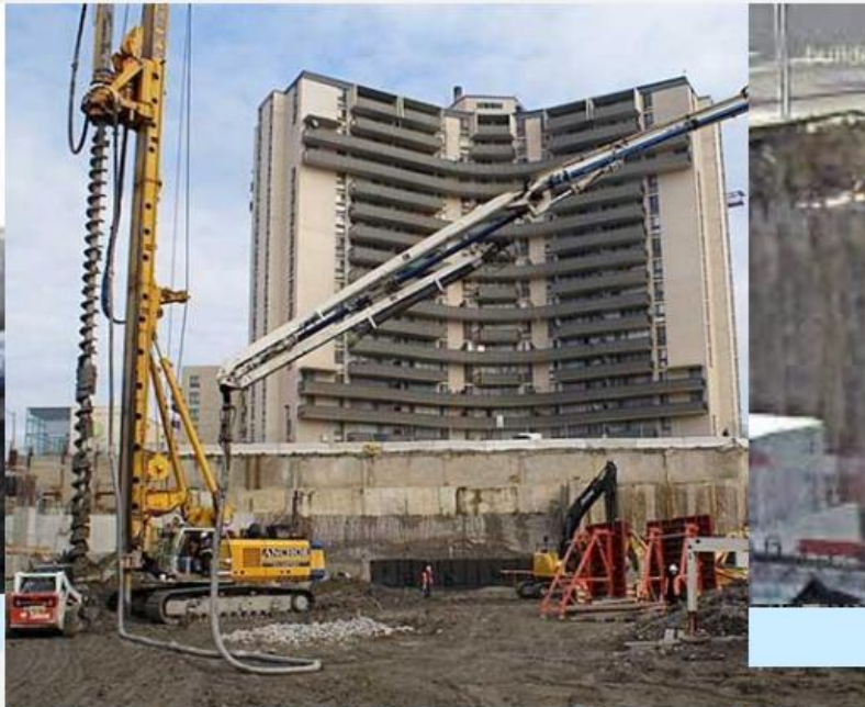
Auger Requires High Headroom to limit Auger Splicing
